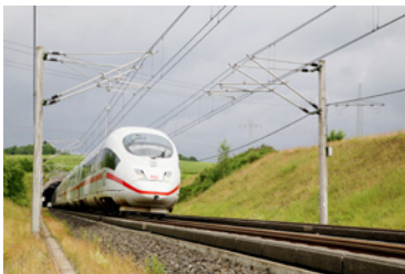
Cover ICE 3 and overhead contact line type Sicat on the high-speed line Cologne – Frankfurt (photo: SPL Powerlines Germany).
