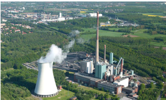
Figure 1: Lünen coal power station of STEAG, view from the northwest (Photo: STEAG).
