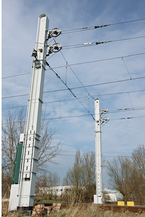
Figure 2: Sicat 8WL5078 tension wheel assembly with mechanical transmission ratio of 1 : 3 up to 24 kN operating load, with integrated weight stack in a H-type pole and installed Sicat CMS contact line monitoring system in the network of the mass transit authority Hallesche Verkehrs-AG.
